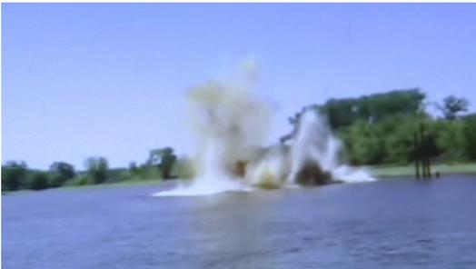
The Corps of Engineers hired contractors to use dynamite to remove the underwater pinnacles south of St. Louis, MO which were obstructing traffic.
