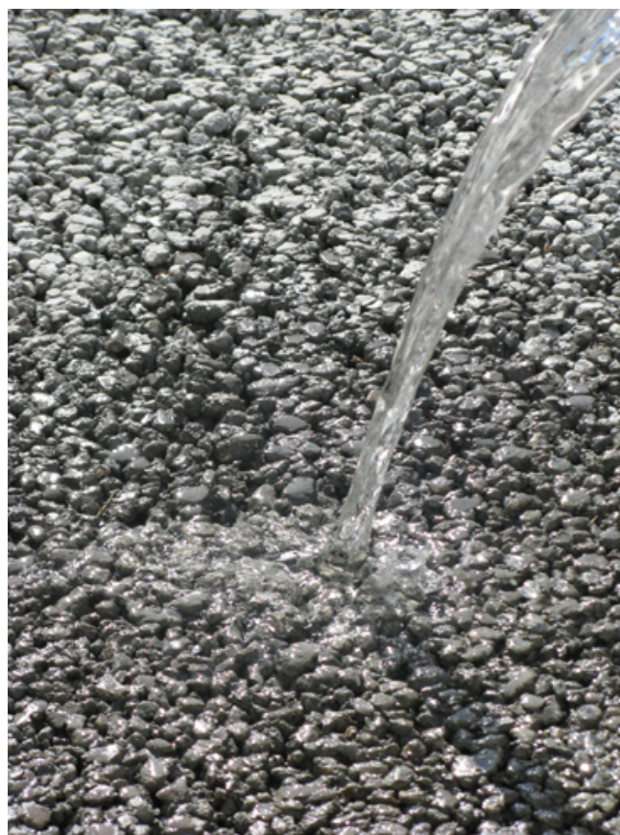
Permeable pavement allows water to soak onto the ground onsite, rather than running off into storm drains that go to the ocean. Karen Setty
